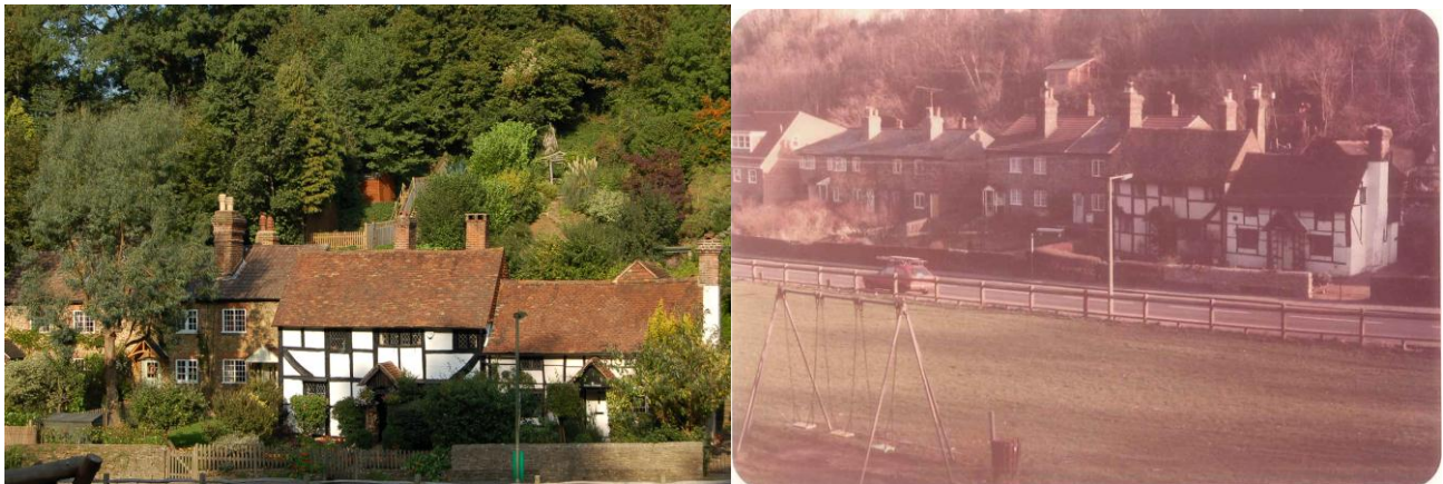
Figure 7: 107- 109 Brighton Road 2014 (left) and in 1984 at the time of designation (right). Comparisons show increasing personalisation and planting of the front gardens which obscures the front of the properties; the loss of the traditional stone wall in front of 107 Brighton Road emphasises the importance of preserving details such as these within the CA.
